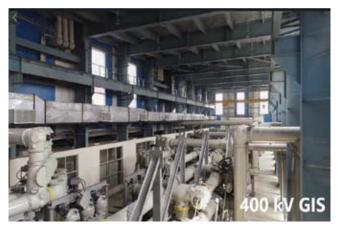
Fig. 1: 400 kV Gas Insulated Switchgear
